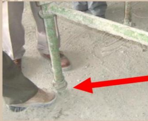
Fig. 4.1 A. Two views of compacted ground or similar soil conditions. Leg located central of mud sill. B. On concrete a base plate is necessary but the mud sill may be omitted.
